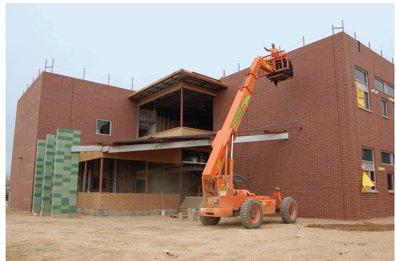
Construction work progresses on the new Aurora Hills Middle School.
